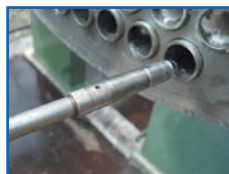
Removal of a hardened polymer from heat exchanger tubes using manually operated waterjetting tools.
