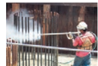
Removing rust from rebar in bridge piling.
