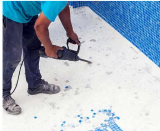
The conventional method of sandblasting, chipping, or jackhammering to remove old pool plaster is an application of the past. These traditional methods of replastering are expensive, ineffective, and cause severe damage to the pool shell.
